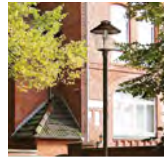
Pedestrian Lighting Columns (5m tall)
