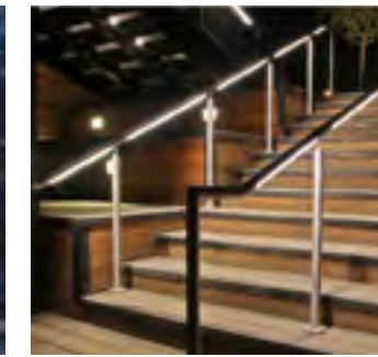
Integrated Recessed Lighting
