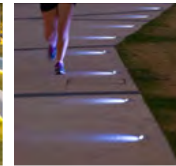
Ground Level Lighting
